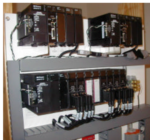
Figure 6 - PLC Based Control System
